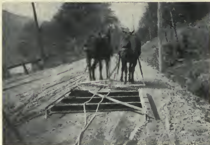
Road maintenance with a steel drag.
